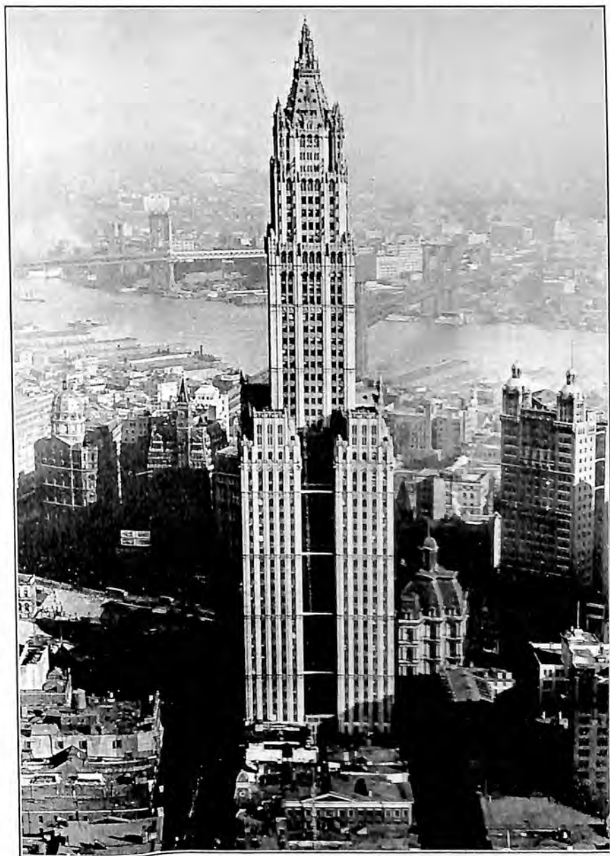
Woolworth Building, New York; Brooklyn and Manhattan bridges in background.—Photo, Hamilton Maxwell.
