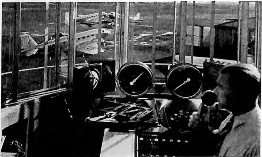
Western Electric Co. Photo
