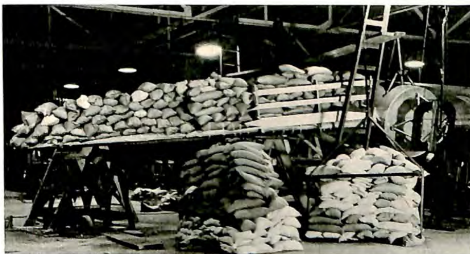
LOAD TEST ON BEEHCRAFT 18
