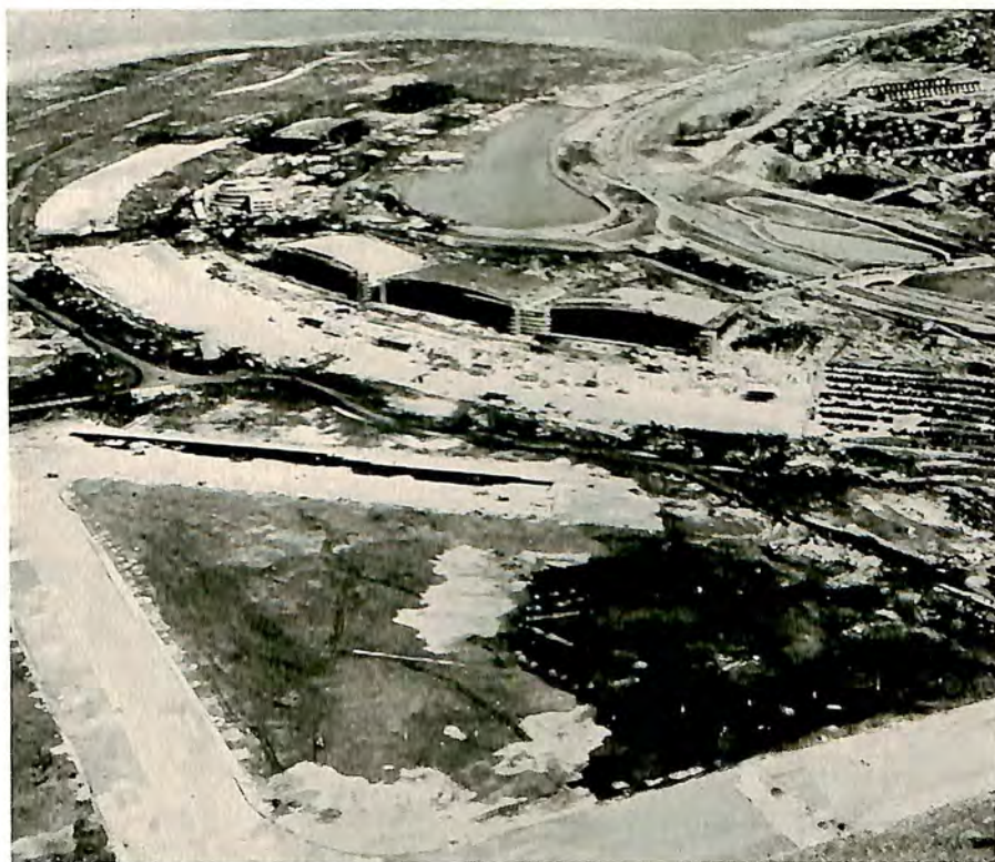
Fairchild Aerial Surveys photo NEW YORK'S NEW AIRPORT
