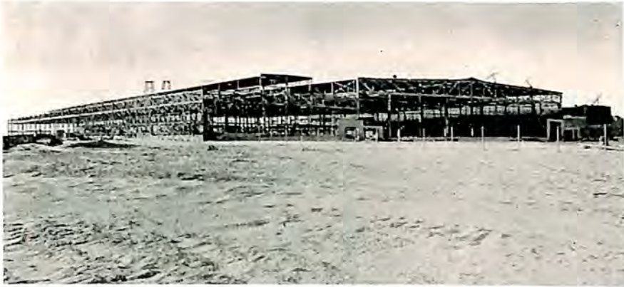
NEW BELL AIRCRAFT PLANT AT NIAGARA FALLS
