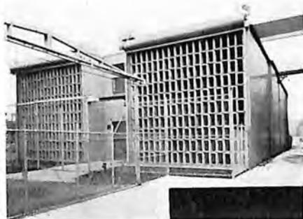
SOUNDSTONE HAS BEEN USED IN ALMOST EVERY AIRCRAFT ENGINE AND PROPELLER TEST CELL.
